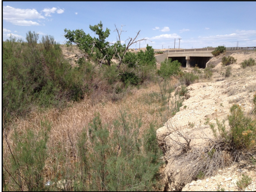
Photo 3 — Wetland WCS-1, looking northwest toward the westbound bridge.
