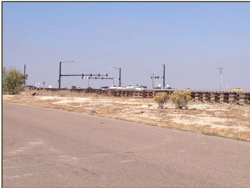
Photo 22 — Looking northwest at the intersection of US 50 and McCulloch Blvd from Dunlap Drive.
